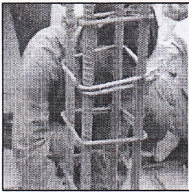
Fig. 1(a): Column Steel Reinforcement
