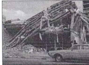
Fig. 8(c): Flat slab Building (Mexico 1985)
